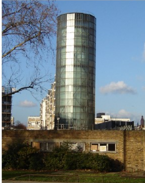
Pimlico District Heating
